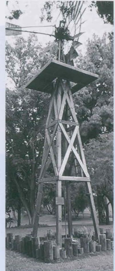
Windmill used to pump groundwater
