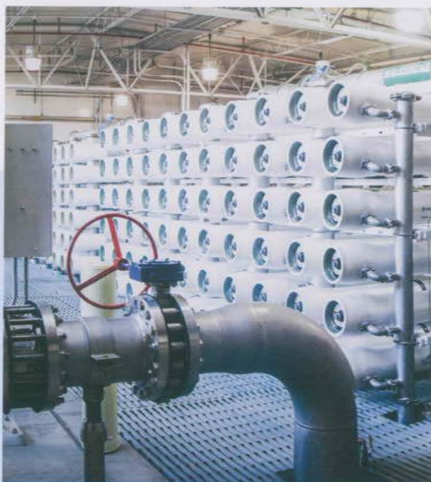
Energy recovery devices are installed at pumps at the Goldsworthy Desalter in Torrance.
