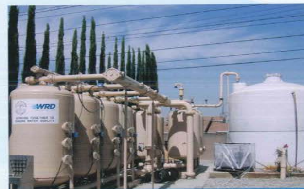
Wellhead treatment system in the City of Paramount
