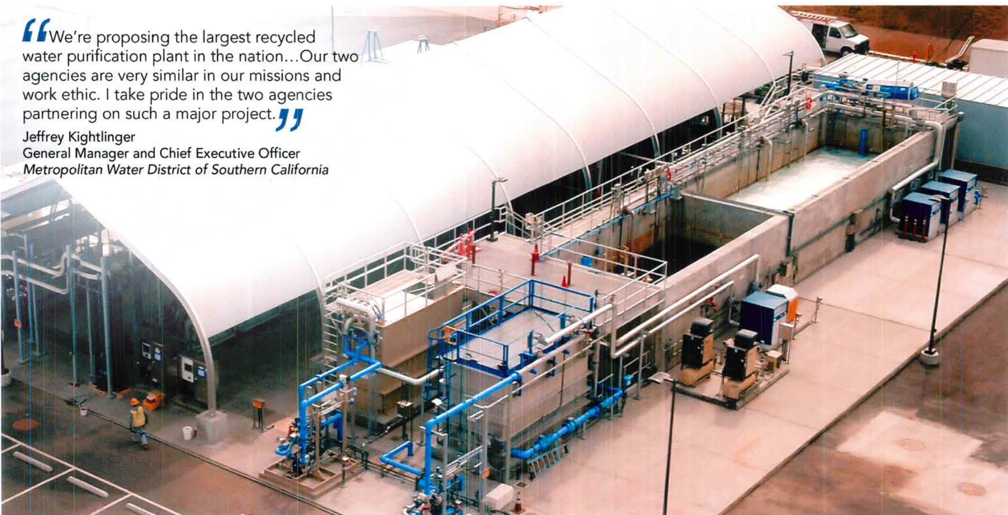
The public is welcome to tour the recently opened demonstration plant and learn how wastewater is being purified. Individual or group tours are available for anyone age 10 and older. The plant uses membrane bioreactors, reverse osmosis and ultraviolet light to remove bacteria, minerals and other chemicals. A full-scale facility would make the region less dependent on imported water.
