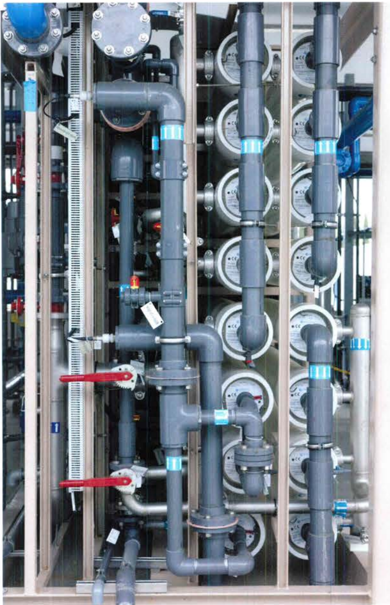
The public is welcome to tour the recently opened demonstration plant and learn how wastewater is being purified. Individual or group tours are available for anyone age 10 and older. The plant uses membrane bioreactors, reverse osmosis and ultraviolet light to remove bacteria, minerals and other chemicals. A full-scale facility would make the region less dependent on imported water.
